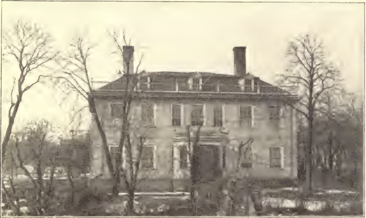
THE SCHUYLER MANSION, ERECTED IN 1761
